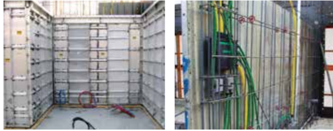
+2 Installation of electrical, plumbing components and steel rebar. Installation of I/C and wall panels
