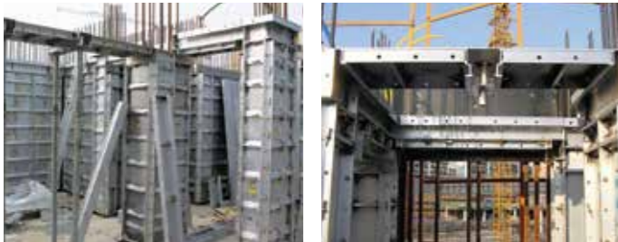
+3 Installation of beam and SC panels
