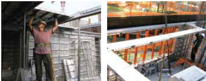
+5 Installation of slab panels
