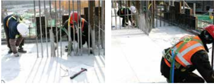
+1 Structural line and level check
