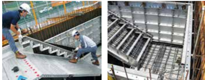
+4 Installation of staircase panels
