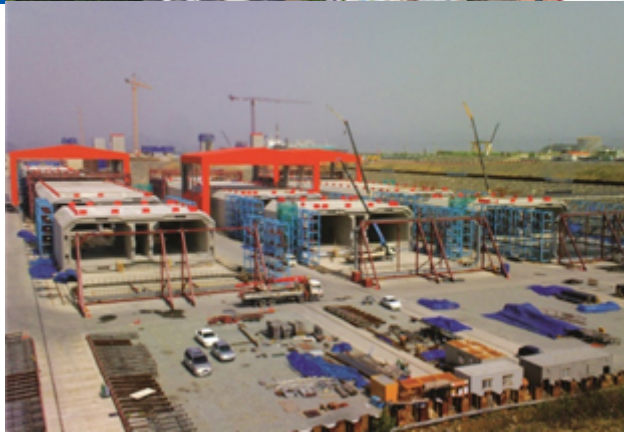
Geoga Grand Bridge (Republic of Korea)
