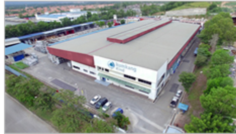
2009. 10 Completed Nilai Factory Malaysia
